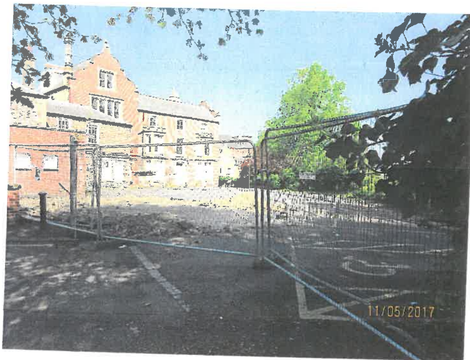
Fencing obstructing path, which should run from the shared use access road (in the foreground of this photograph) to the sign just visible in the centre of the photograph (right hand corner of Prospect House)
